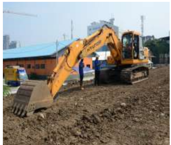
Lomba Operator Excavator
