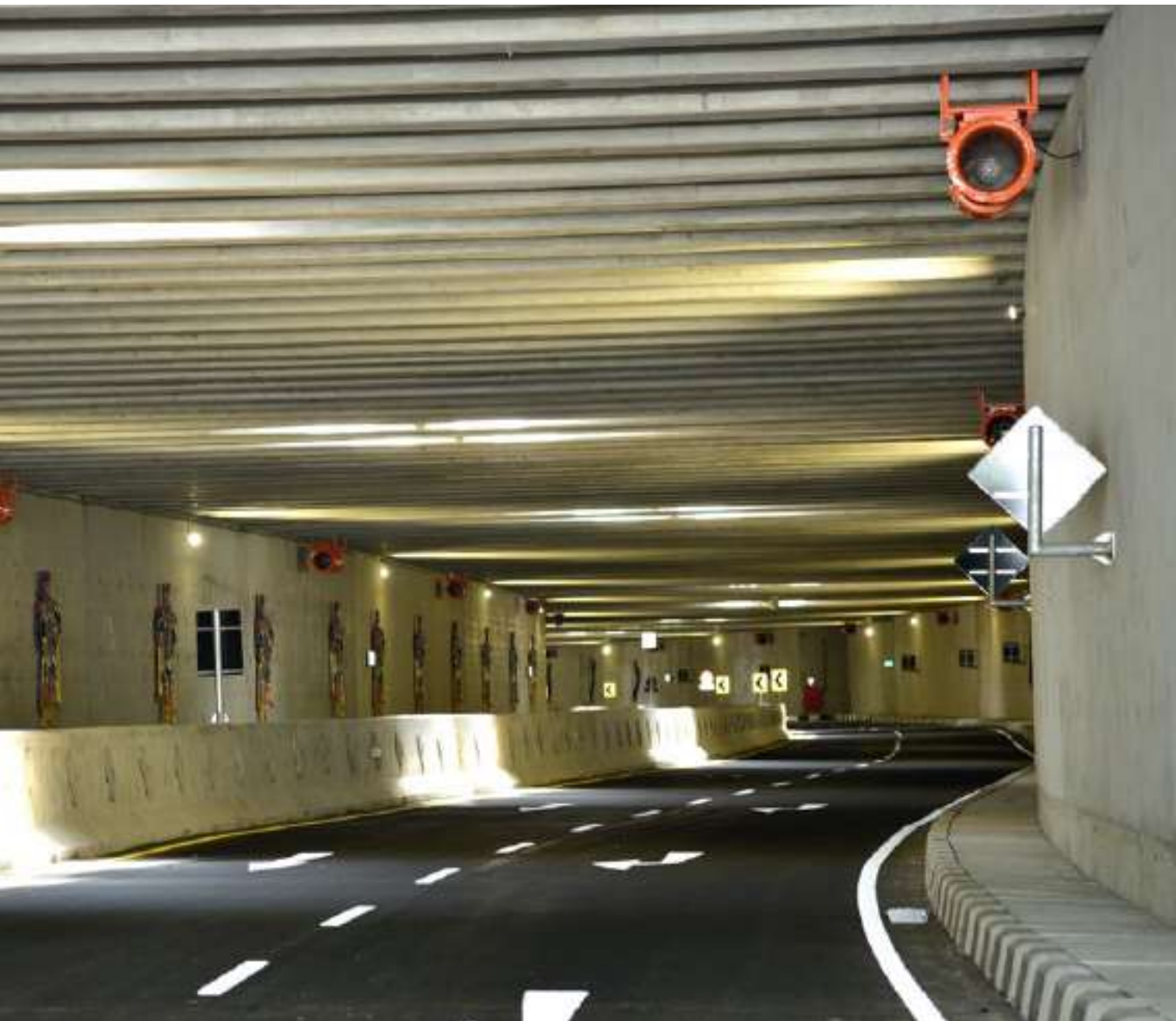
..... Underpass NYIA New Yogyakarta International
