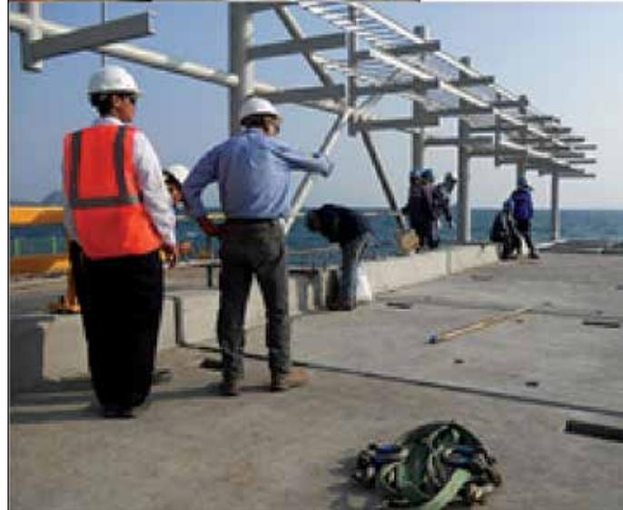
**PROSES PENUMPUKAN DAN PERAKITAN SLAB PRECAST KE STEEL STRUCTURE**
