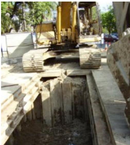
Gambar 14. Shaft Excavation
