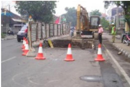
Gambar 13. Deck Cover Excavation
