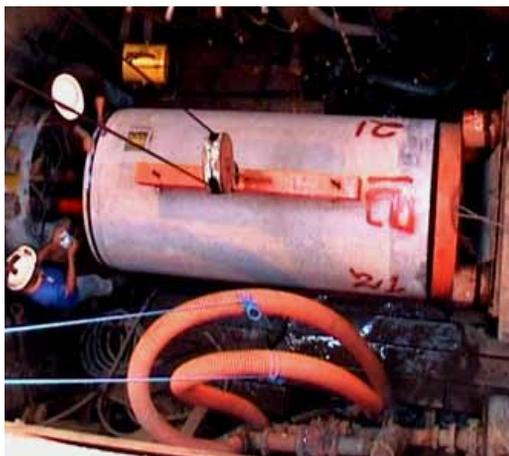
Gambar 10. Install Pipe Jacking
