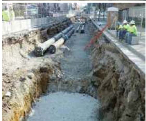
Pengerjaan Proyek Galian Konvensional (Sumber: http://nashvilledistrictenergy.com/dt_gallery/music-city-convention-center-service-lines-installed/opentrenchfacingeast/ )
